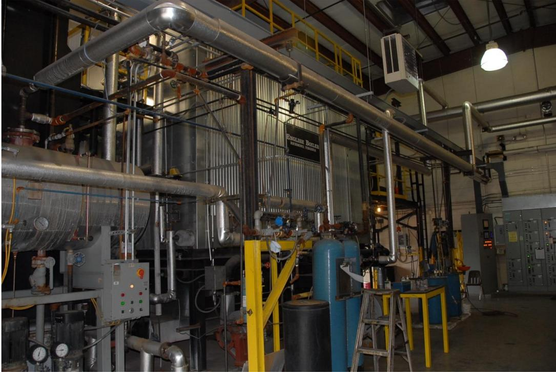
Figure 5. Rõnile's 400 HP English Boiler generates process steam for the 350,000 square foot manufacturing facility.
