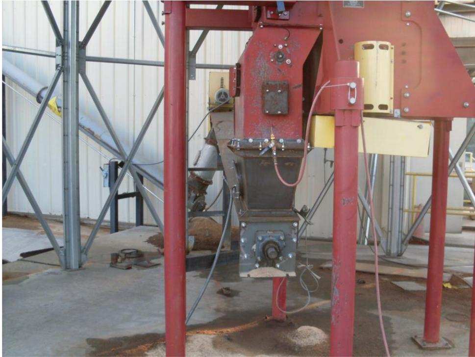
*Figure 3. Rönile's handling system that conveys fuel from the storage silo to the day bin.*
