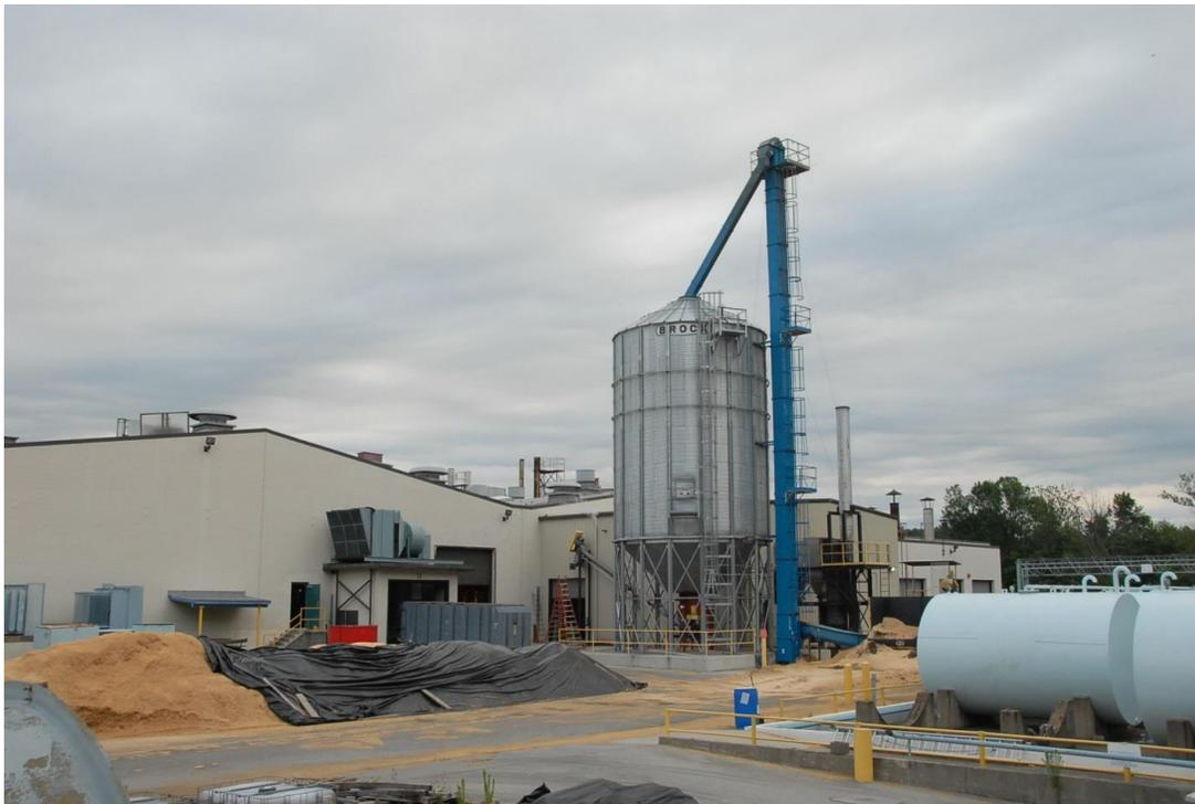
*Figure 4. Rönile's external biomass handling and storage system.*
